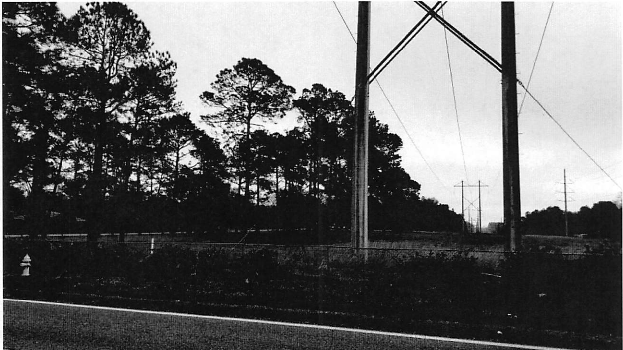
Subject site along Schindler Drive Source: Staff, Planning and Development Department Date 02.24.17
